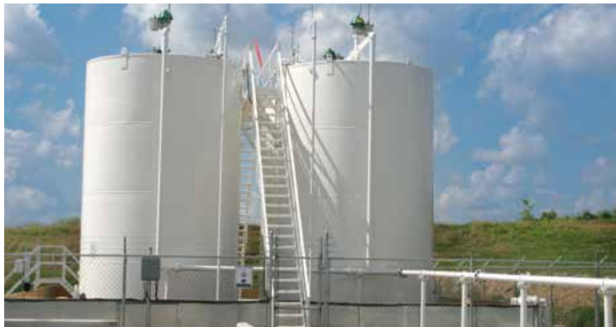
Image 2. In-the-field storage tanks are used to house raw crude oil and natural gas before it can be transported for refinement. Operators must control the amount of potentially harmful vapors that are released to the atmosphere from the tanks and are turning to VRUs as a solution.
